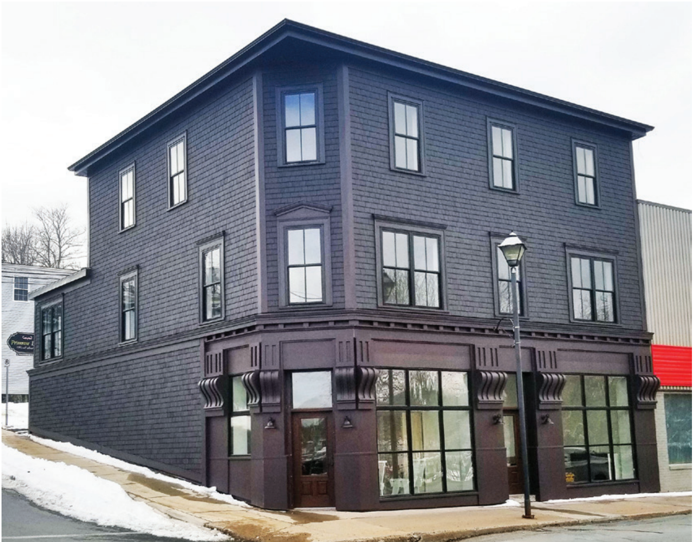
The rehabilitated Rofhe Building in February 2021 (photo courtesy of the author)
