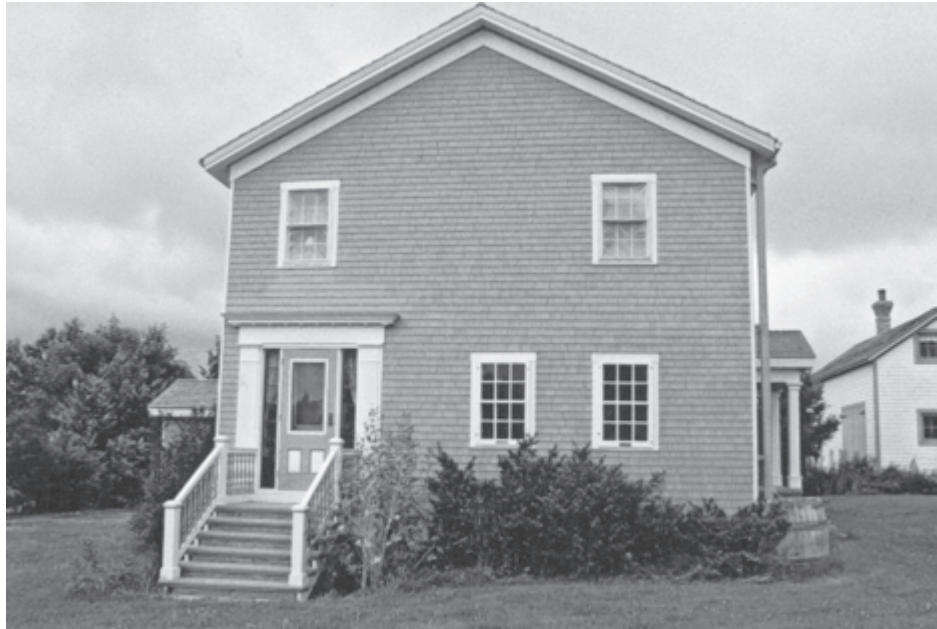
Note the Greek revival doorway leading into the main part of the house from the side. Approached from this angle it could be mistaken for a main entrance.
