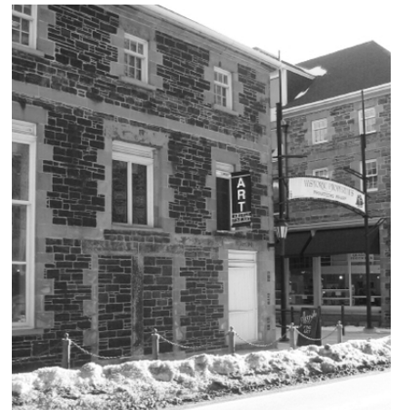
The Collins Bank Building, Upper Water Street, Halifax.
