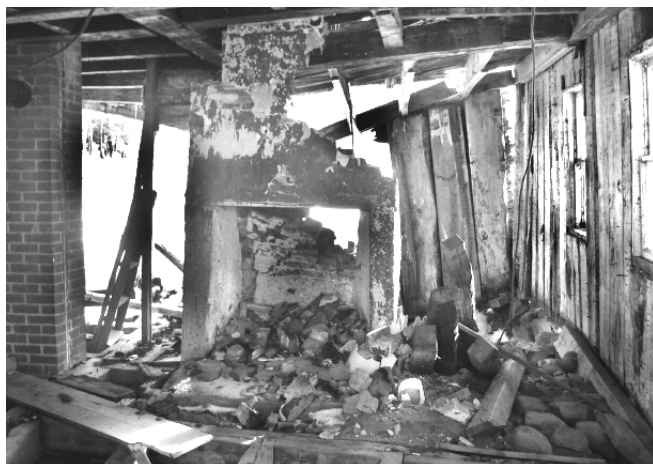
Construction details are exposed in 2009. (Peter Delefos)
